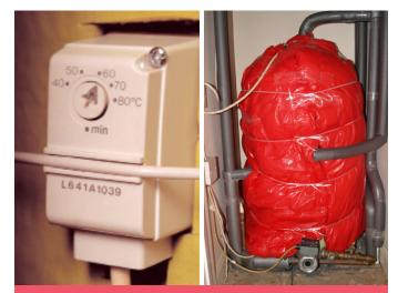
A cylinder thermostat (left) will stop you wasting money on overheating your water, while to save more on water heating, make sure you get your hot water cylinder and pipes insulated too
