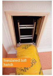
draught-excluding material around the edge of the frame. If matting or rigid insulation boards have been used for insulating the loft, any cut offs could be used to insulate the hatch. It is also important to make sure that the loft has adequate ventilation. Colder air is more likely to form condensation which can lead to damp problems.
