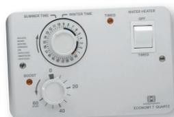
Make sure the 24 hour clock is correct against the winter-summer line (based on the time of year), otherwise it may heat up during on-peak hours. For extra hot water during the day turn the boost dial, and the immersion will switch off after the selected period of time.
